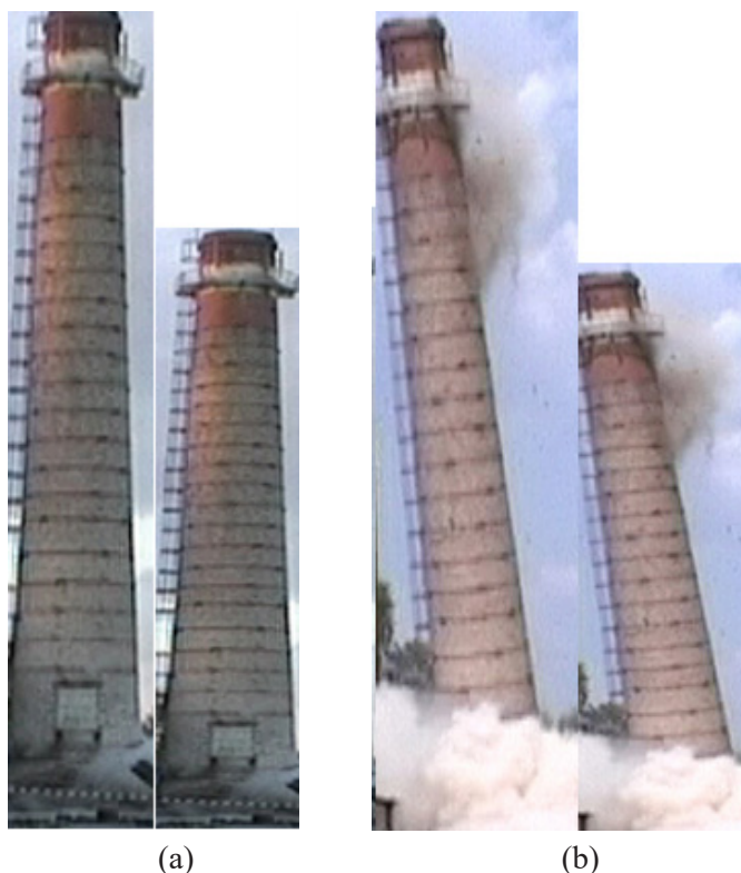
Figure 1. Photographic recording of anthropogenic civilian destruction of two brick chimneys
